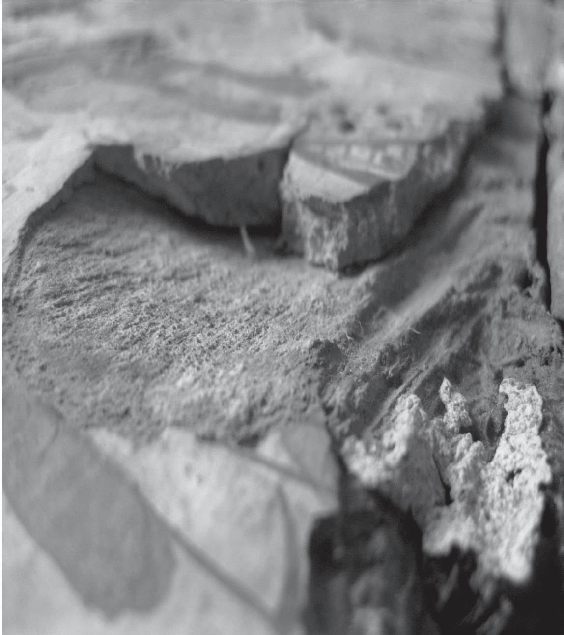
Photo 6: A detail of the area where the gesso is thickened due to the irregular surface of the composing planks
